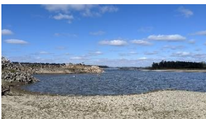
Len small levee breach.
