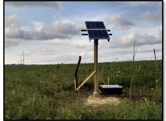
Grand River Grasslands, Ringgold County IA. Installed phenocam with solar panel and battery.
