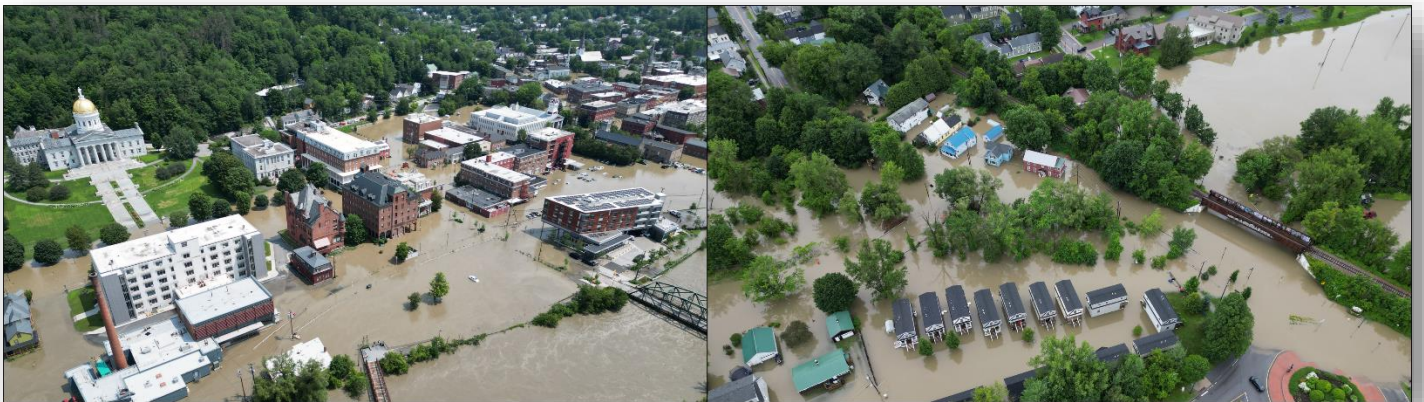
The flooding devastated Vermont's cities, towns, and villages near waterways. Homes and businesses were inundated with water, resulting in millions of dollars' worth of damage. VermontView's drone teams captured the impact.
